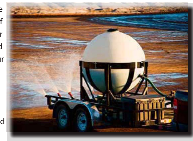
SILICATE COATING SUBSTITUTE FOR ASPHALT SURFACE
